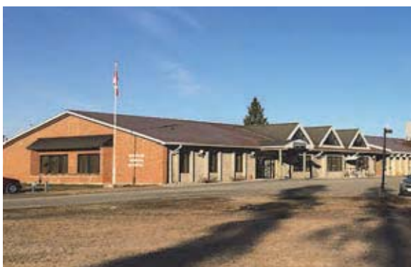
Atikokan General Hospital’s renovated space will provide integrated acute and long-term care for the community.
